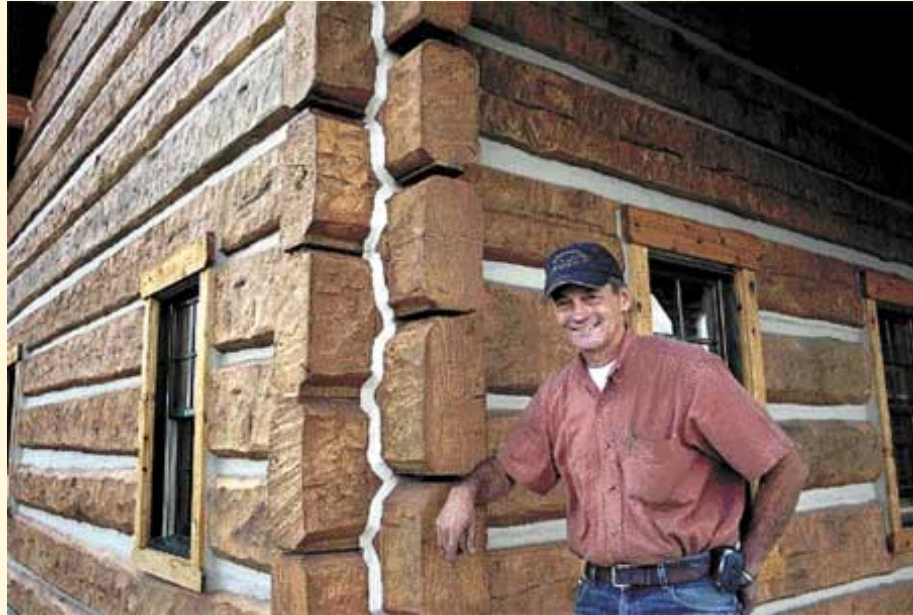
Dick Morgenstern stands in front of his office made of cultured concrete logs. The logs of concrete look like they're made of wood. Photo by DEAN BAKER/InBusiness
